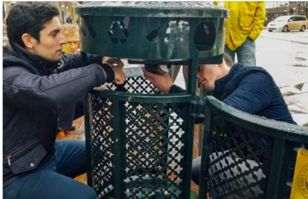
Employees of Nordbarnes install a smart sensor in a trash bin at Sixth and Market streets in San Francisco in 2016, during a trial of the smart trash system. The smart sensors will be installed in 1,000 trash bins around the city starting in Spring 2018. (Courtesy of San Francisco Public Works)
